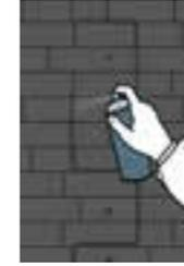
The spray is used to balance colours between joints and panels. So once the paint is dry spray over the joints one flash at a 40cm distance
