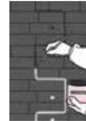
When the putty is dried paint the joints where putty was previously applied using different brushes
