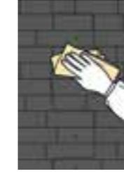
Right after when the paint is still wet rub a wet cloth over the joints to cover the pores. Do it as many times as needed.
